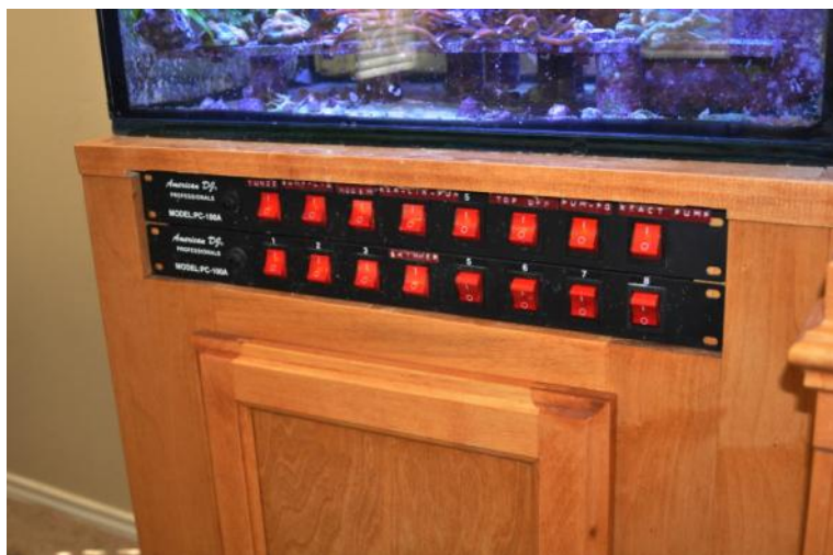
DJ switch panel
